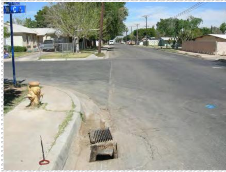
Photo 2-1: Existing catch basin as part of combined system
