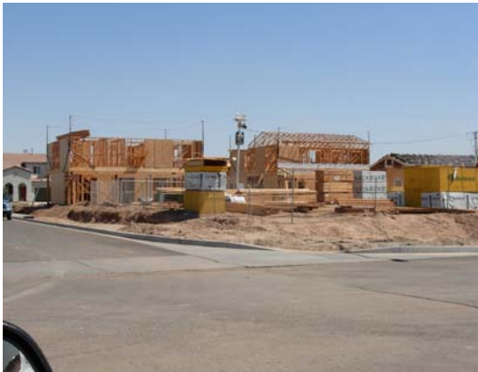
Single-family Homes under Construction
