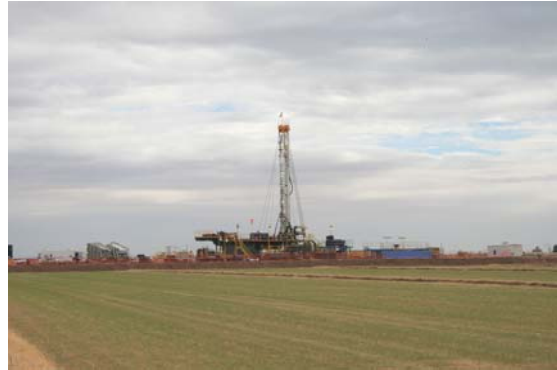
Geothermal Energy Well
