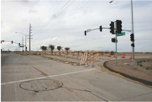
SR-111 Bypass Construction
