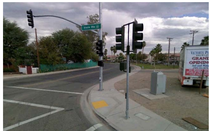
Pedestrian push button at the intersection of Brawley Avenue and Malan Street.
