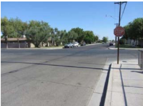
The intersection of 1 st Street and A Street lack crosswalks.
