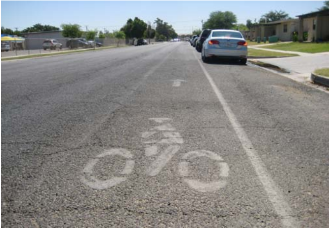
The existing bicycle network in Brawley consists of Class II lanes.
