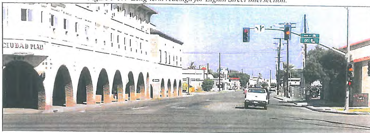
Excess width on Eighth Street that can be closed in with curb extensions.
