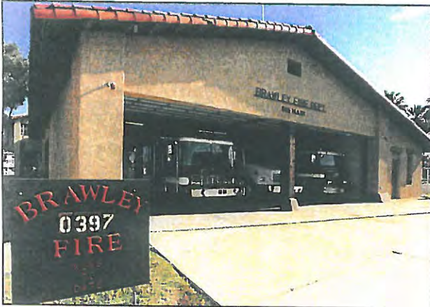
Brawley Fire Department headquarters.
