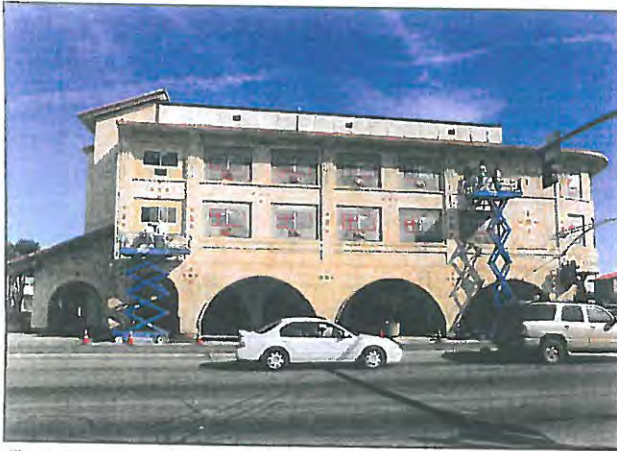
Current renovation in progress in Brawley.
