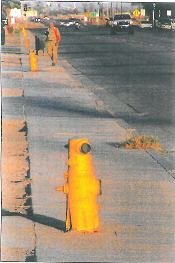
Pedestrian and wheelchair obstacles on sidewalks.
