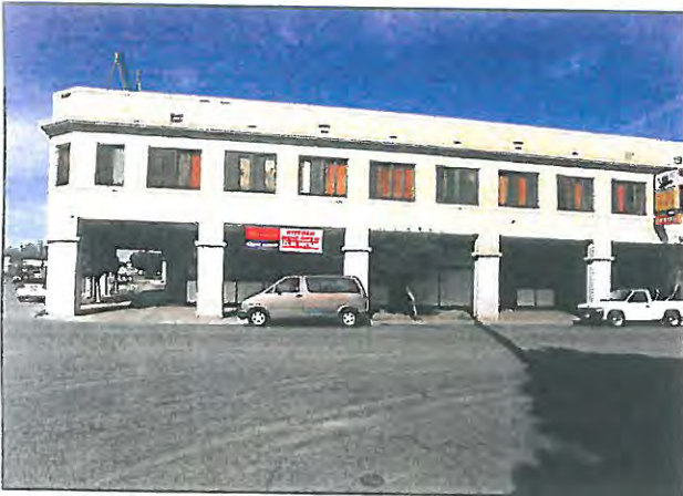
Another potential opportunity for renovation.
