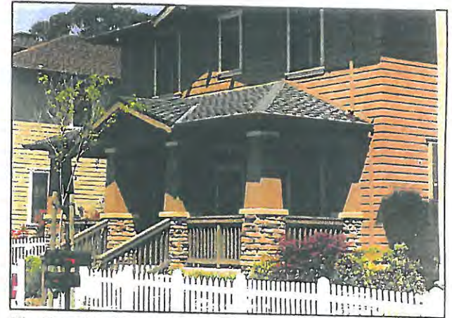
The Hercules, CA code specifies every architectural detail.
