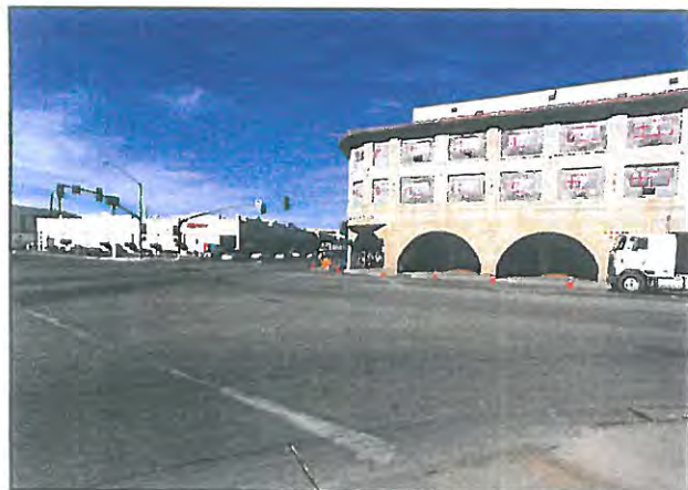
Pedestrians feel vulnerable in exposed crosswalks.
