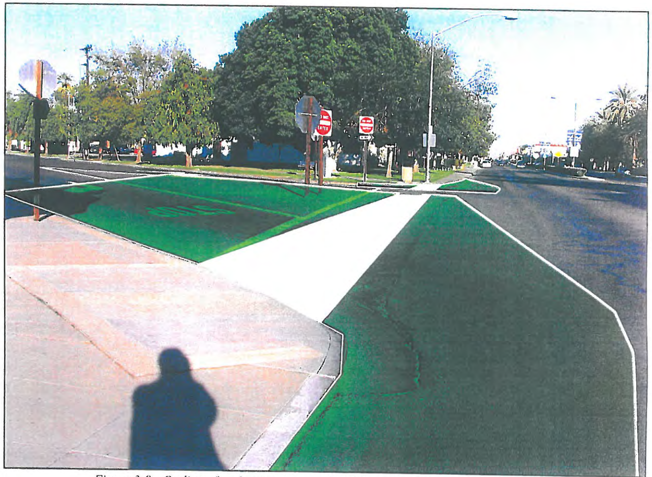
Figure 3-9: Outline of curb extensions on West Plaza corner near the Police Station.
